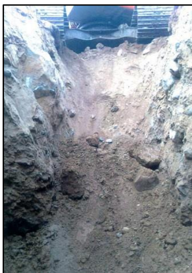
Photo 3: Collapsed subsoil
